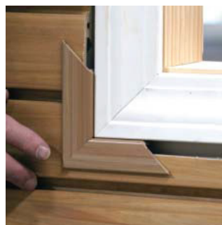
Flat, Narrow L, Wide L and Large L trim can be used in combination.
