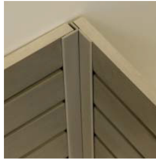
Attach Flat to panel with the edge against the Narrow L or Wide L Trim.
